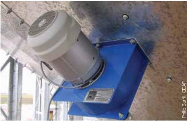
Aeration fans fitted to silos can rapidly reduce grain temperatures.
