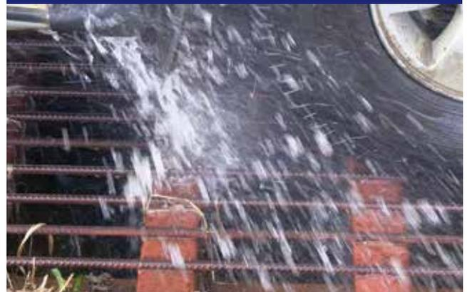
If possible, install a sump to collect waste water and debris.
